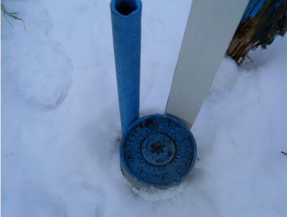
Picture 5 –Found Berntsen, 1 Inch Iron Pipe and Wood Post
