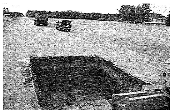
Dig looking East
