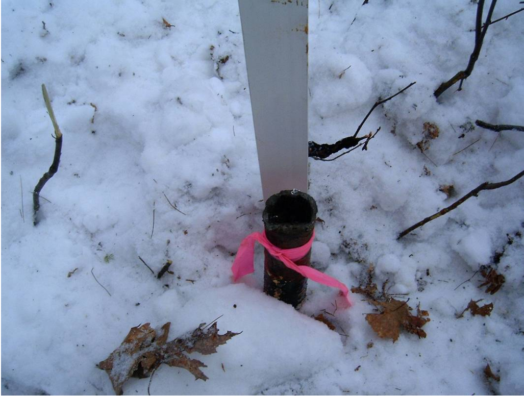
Picture 5 –Found 1.5 inch Iron Pipe at Corner
